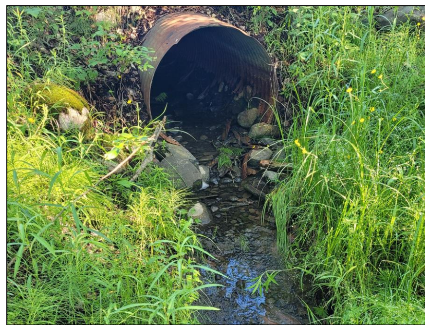
Photo. 10: Culvert conveying flow from site to east of rail line, June 28, 2023
