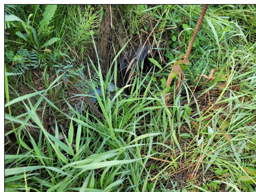
Photo. 6: Culvert conveying flow east of Falcon Street, June 16, 2023.
