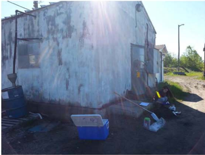
Site 1 – Fuel Storage Shed and sampling pit
