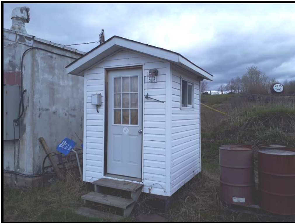
PHOTO # 2 Fuel Off-loading Shed (small)
