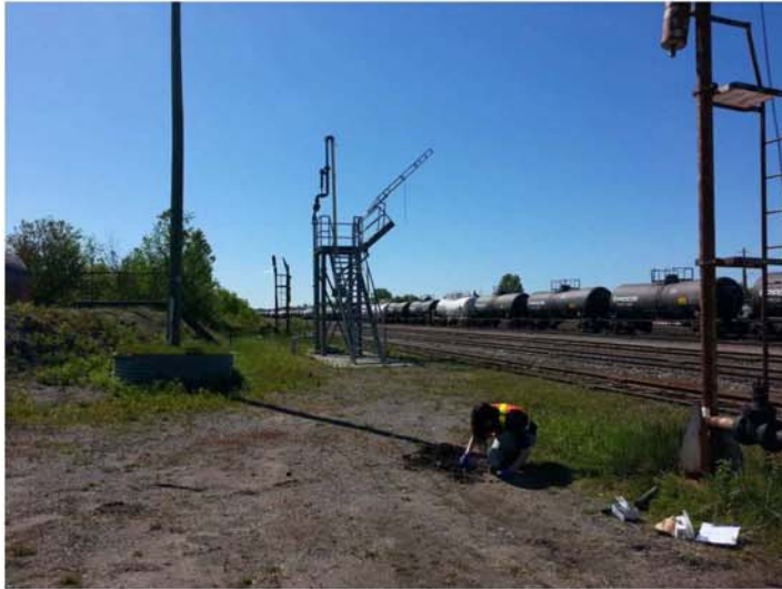
Site 3 – North Offloading Crane and sampling pit
