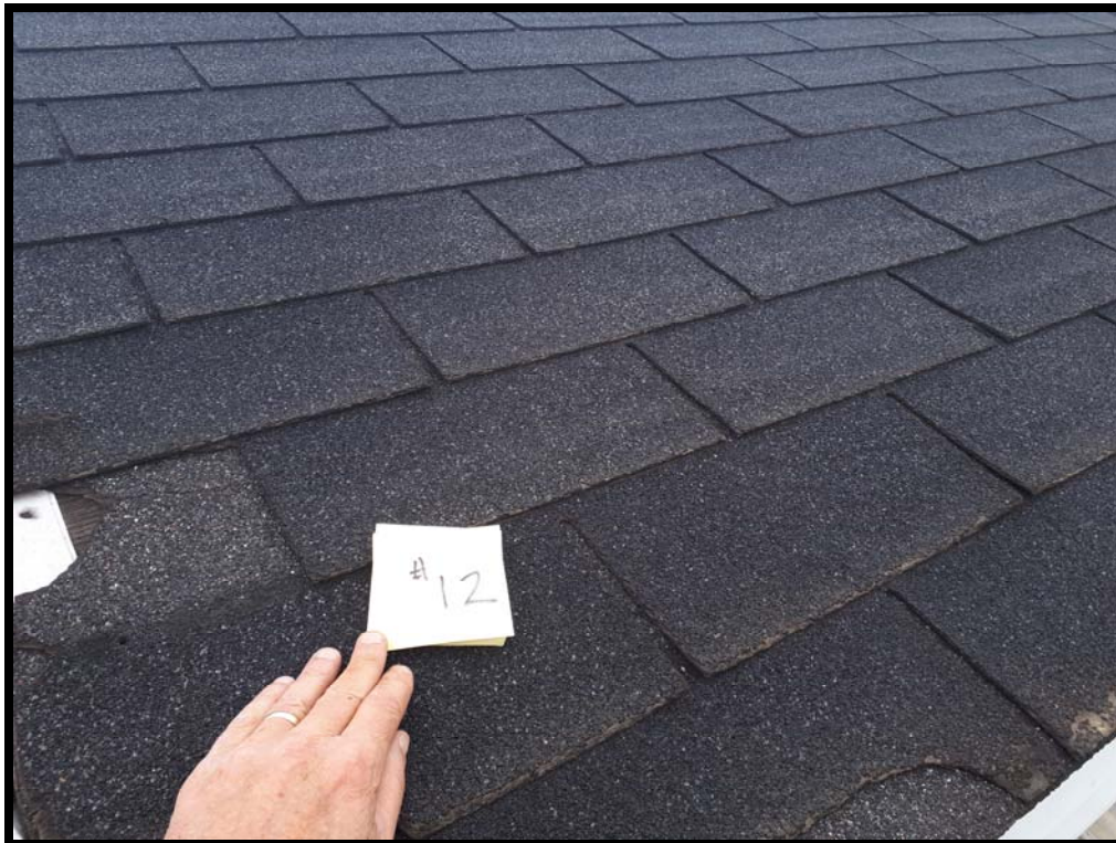
PHOTO # 10 Sample # ONR 12 : Non-asbestos tar roofing shingles on fueling shed.
