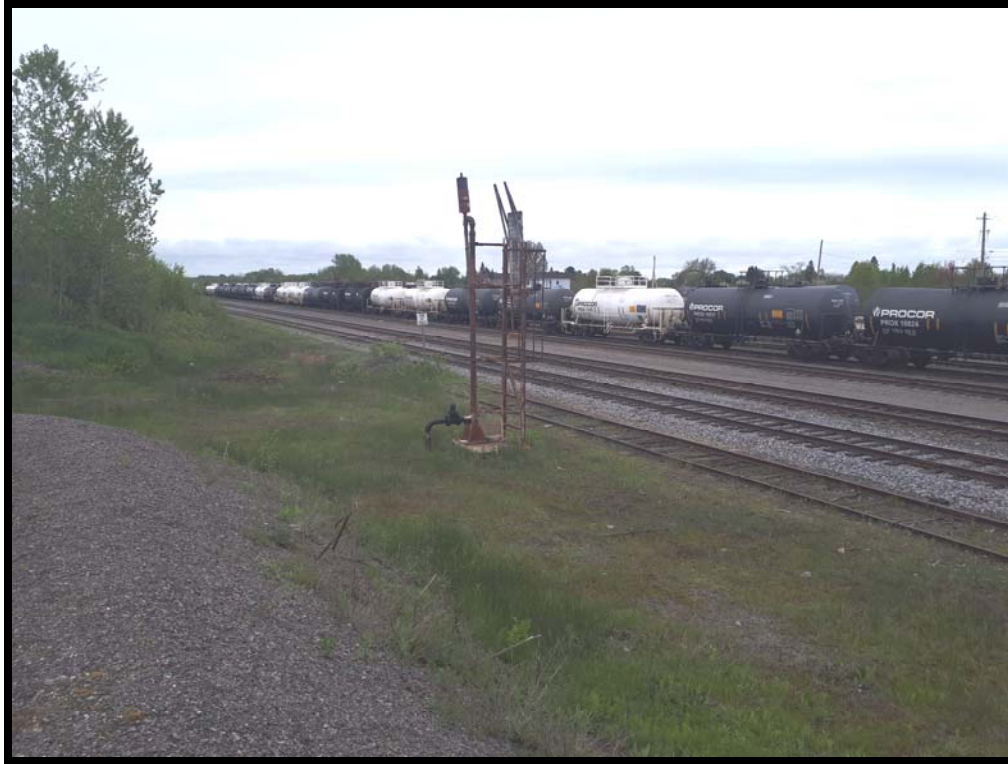
PHOTO # 3 "Old" Fuel Off-loading Cranes (2)
