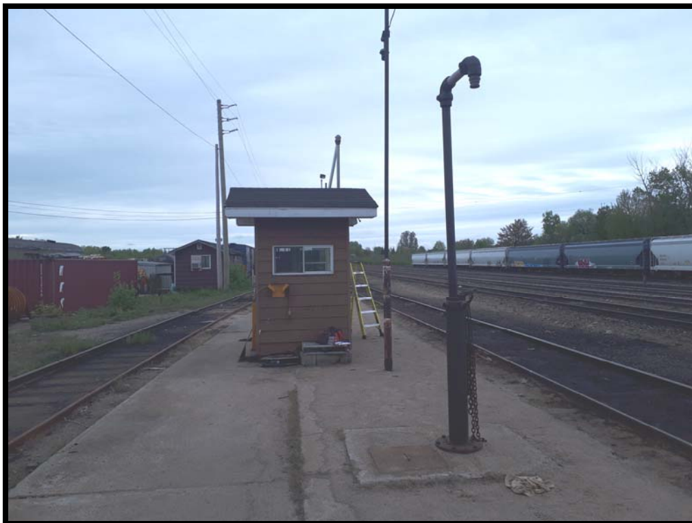
PHOTO # 6 Fueling Shed
