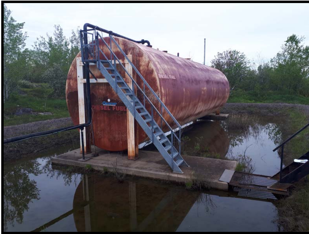
PHOTO # 5 Fuel Storage Tank (Diesel)
