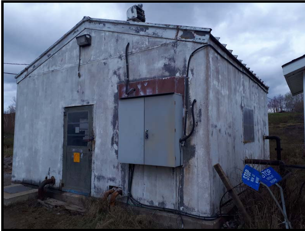
PHOTO # 1 Fuel Off-loading Shed (metal)
