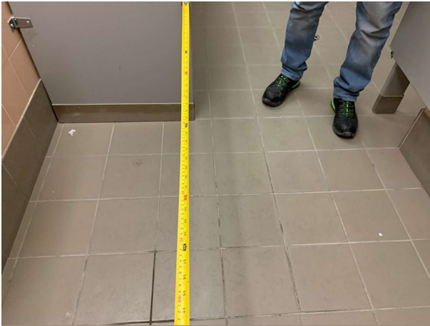
Photo 43 – Clear turning space diameter within the stall
