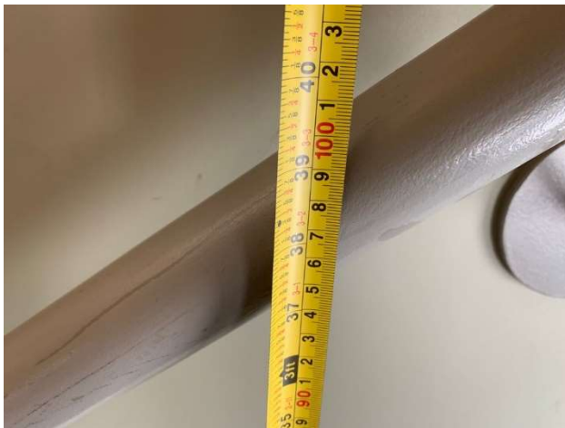
Photo 71 – Height: Side Handrail
