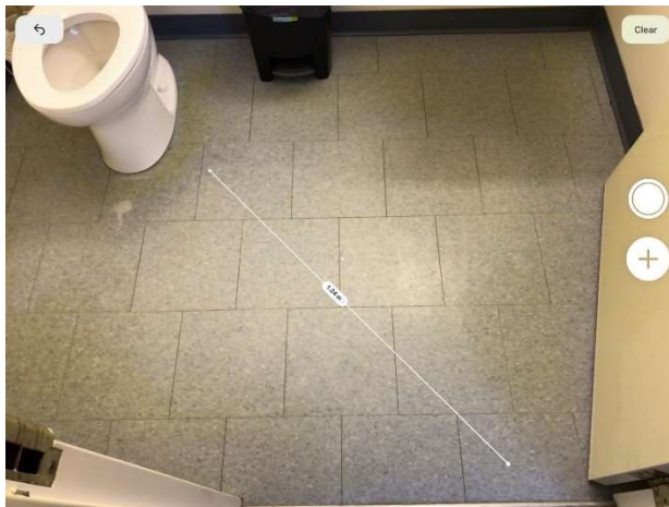
Photo 29 – Shower stall space
