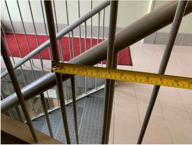
Photo 73 – Size of guard openings
