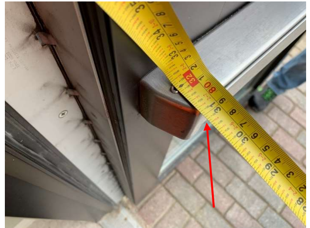
Photo 4 – Main entrance door - clear width of open door
