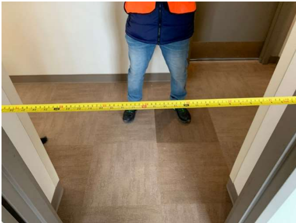
Photo 21 – Interior Door-Clear width of open door
