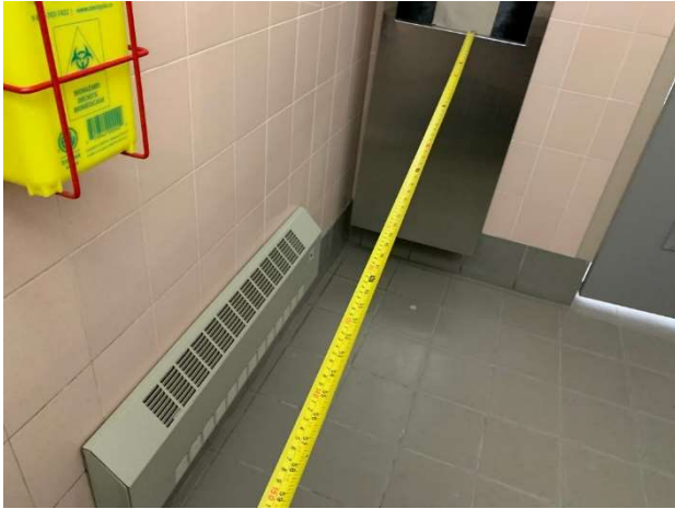
Photo 55 – Horizontal distance from the edge of the lavatory
