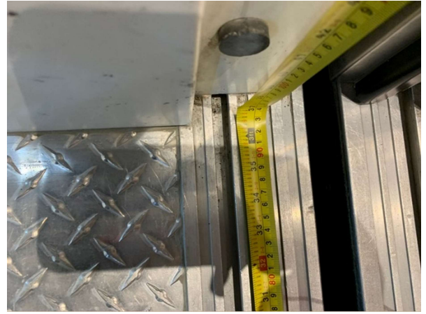
Photo 80 – Door clear width (close-up measurement)
