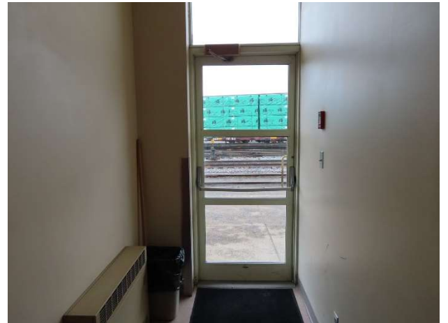
Photo 12 – General view of corridor from offices to entrance to the shops
