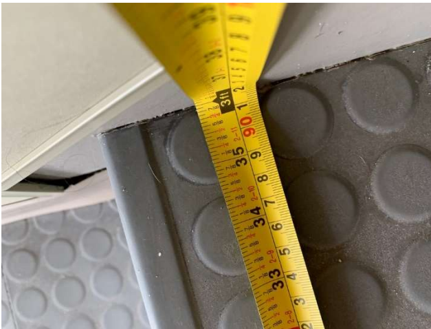
Photo 69 – Clear Width (close-up measurement)
