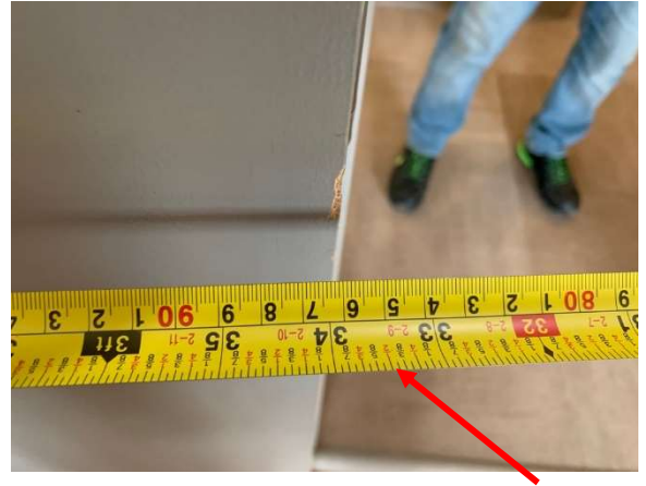
Photo 28 – Clear width of open door
