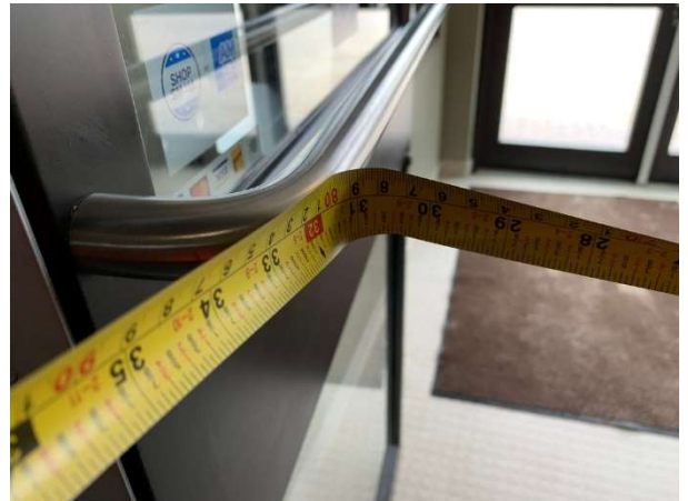
Photo 18 – Inner Door: Clear width of open door
