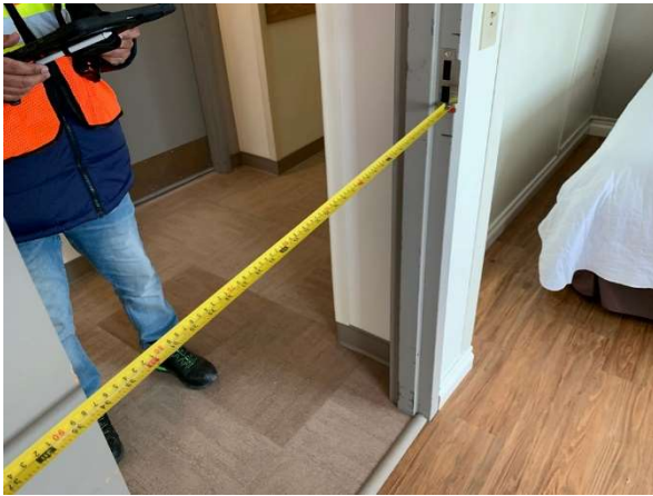
Photo 27 – Clear width of open door
