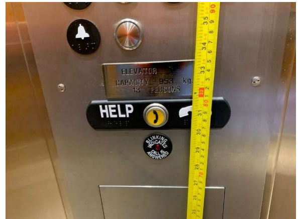
Photo 86 – Distance between center line of emergency control buttons and floor
