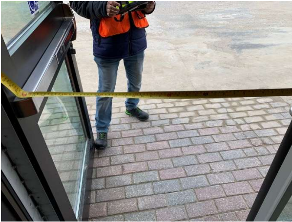
Photo 15 – Outer Door: Clear width of open door
