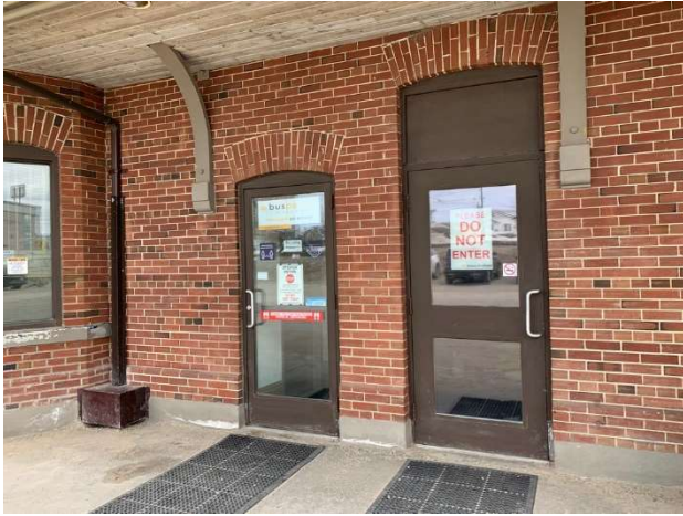
Photo 7 – General view of hotel entrance door - Pull side
