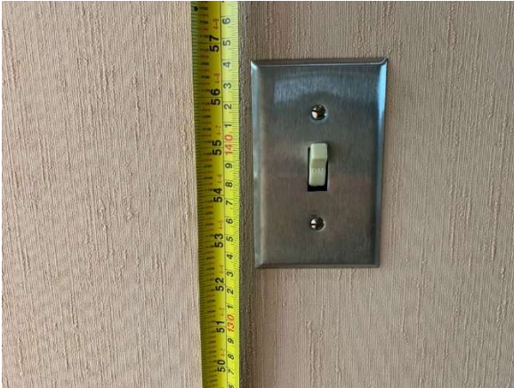
Photo 91 – Height of controls
