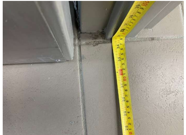
Photo 36 – Interior Door - Clear width of open door (close-up measurement)
