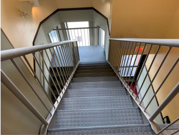
Photo 67 – General view of interior stair
