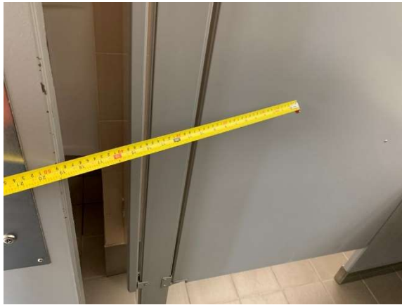
Photo 45 – Clearance between outside of stall face to in-swinging washroom door
