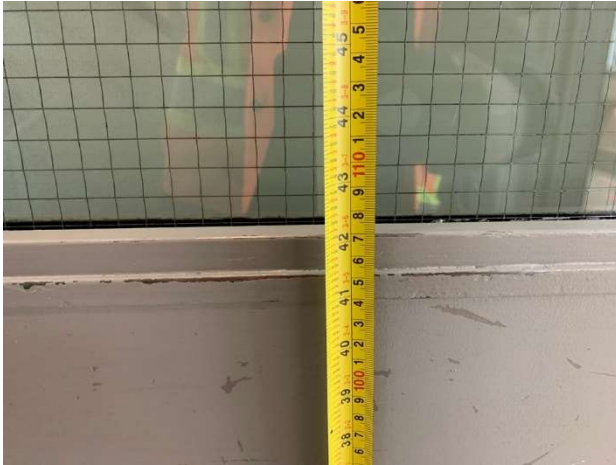
Photo 37 – Interior Door - Distance between bottom of vision panel to floor
