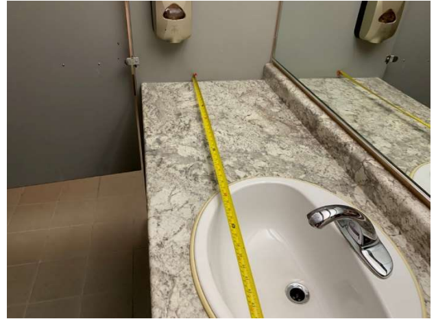
Photo 56 – Distance from the front of the lavatory
