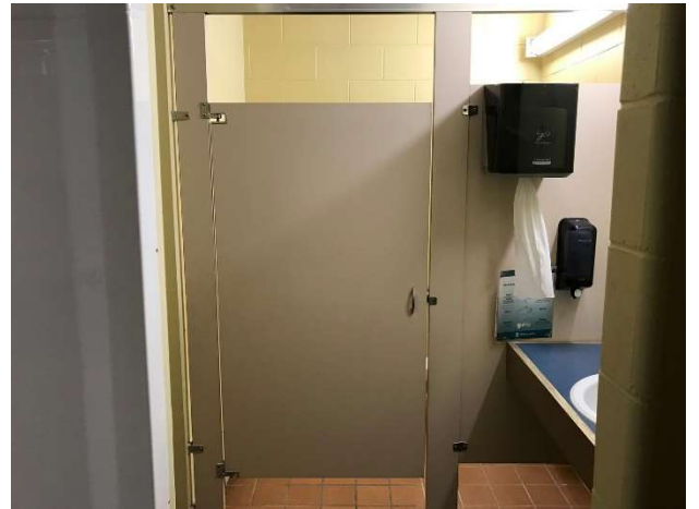
Photo 40 – Height of towel dispenser from finished floor
