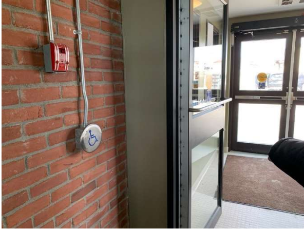
Photo 19 – Inner door: Control located so that the path of travel is obstructed
