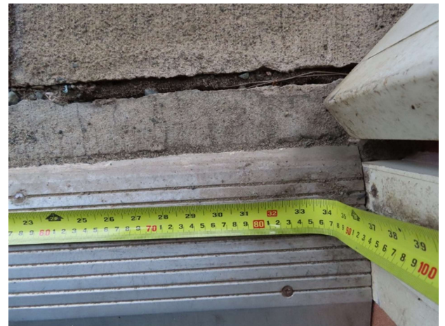
Photo 6 - Clear open door width of exterior door (closeup)
