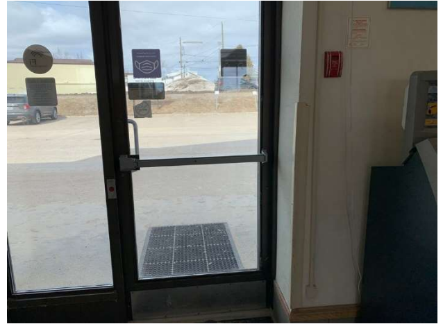
Photo 2 – General view of main entrance door – push side
