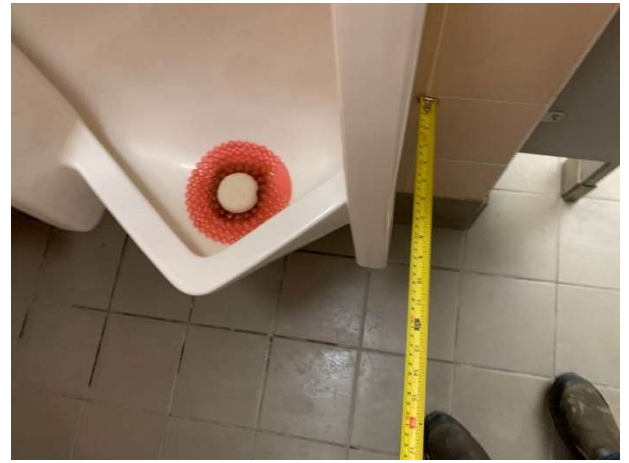
Photo 50 – Depth of the urinal from the outer face of the rim to the back
