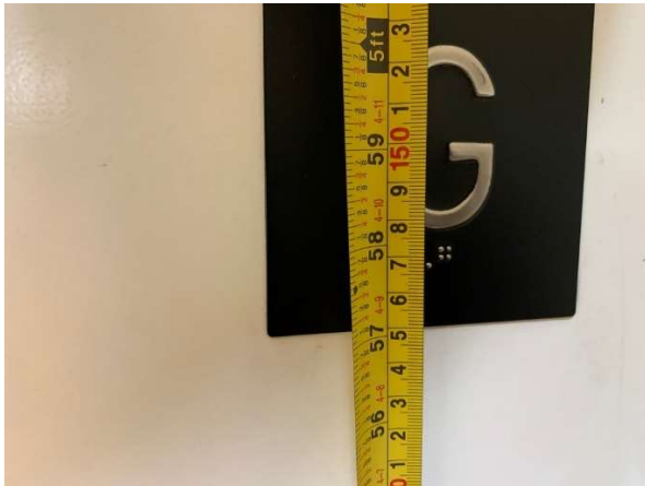
Photo 87 – Distance between baseline of characters and floor
