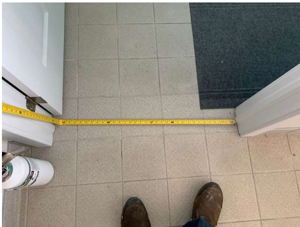
Photo 41 – Station Office Solid Door: Clear width of open door
