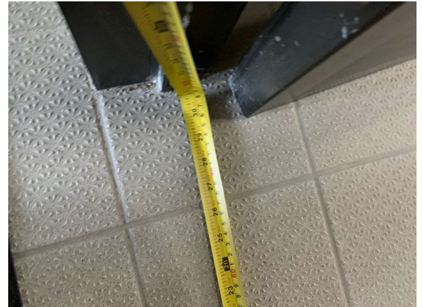
Photo 40 – Ticket Office Transition Door: Clear width of open door
