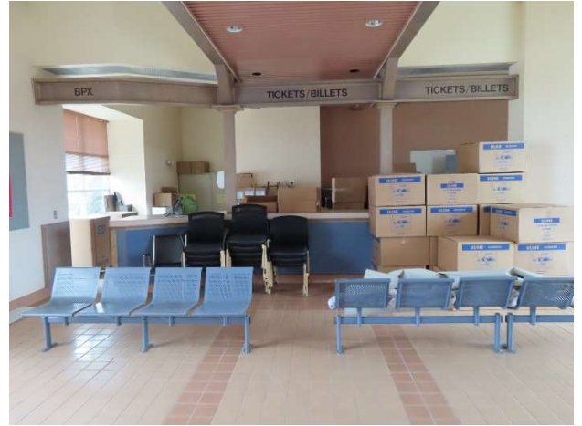
Photo 56 – Height of towel dispenser from finished floor
