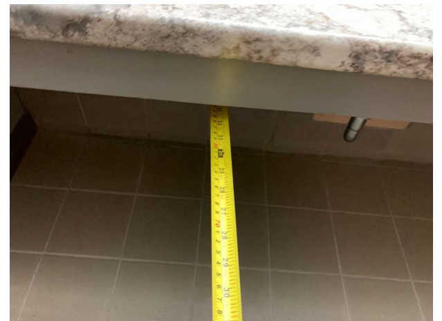
Photo 54 – Depth of floor space under lavatory
