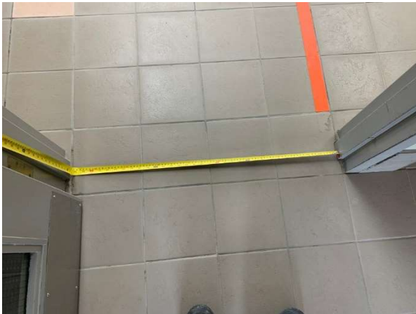
Photo 35 – Interior Door - Clear width of open door
