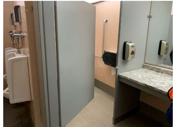
Photo 46 – General view of accessible stall
