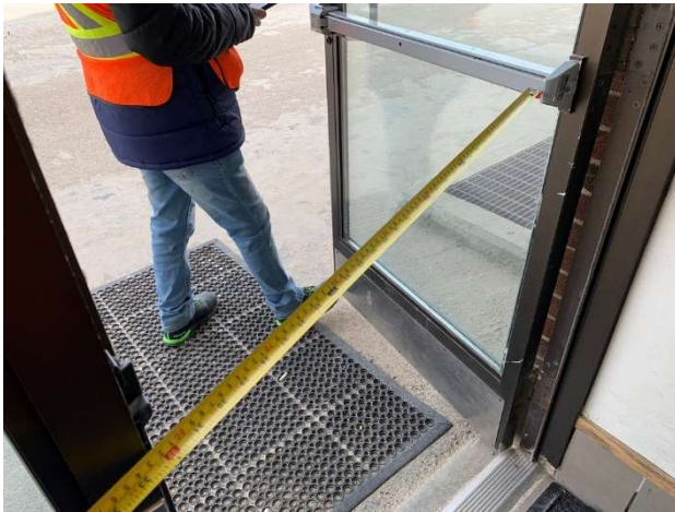
Photo 3 – Main entrance door - clear width of open door
