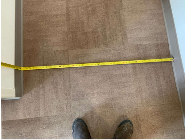
Photo 25 – Wheelchair turning diameter in open space
