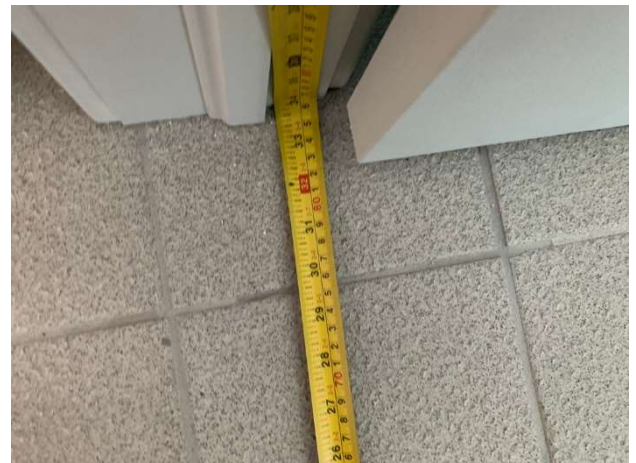
Photo 42 – Station Office Solid Door: Clear width of open door
