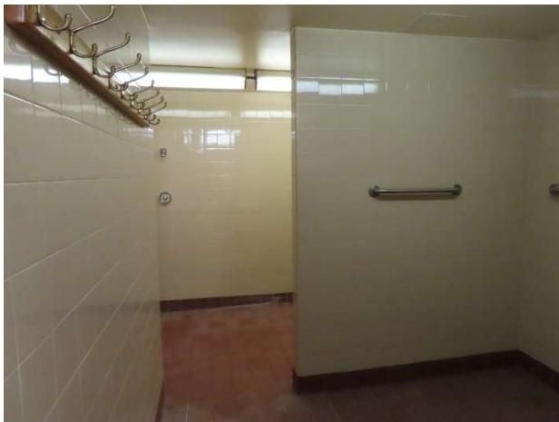
Photo 35 – Height of thermostat finished floor
