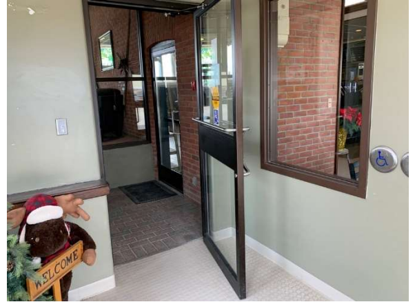
Photo 20 – Outer door: Control located so that the path of travel is obstructed
