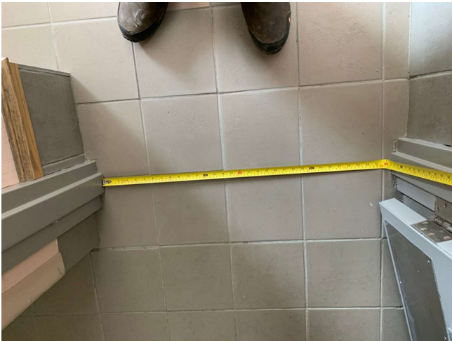
Photo 57 – Entrance Door opening width
