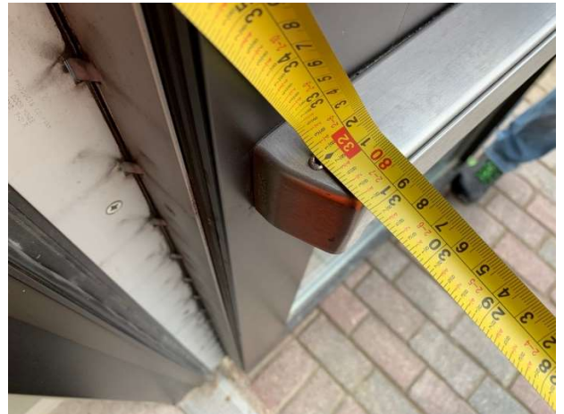
Photo 16 – Outer Door: Clear width of open door (close-up measurement)
