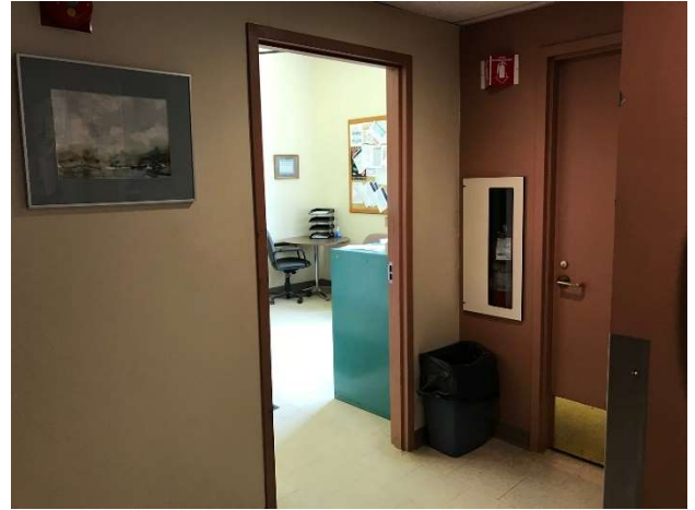
Photo 20 – Insufficient space within the individual washroom
