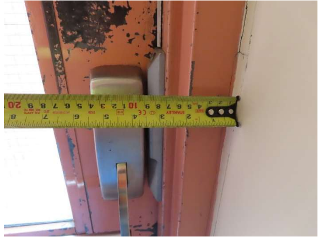
Photo 4 - Location of exterior door
