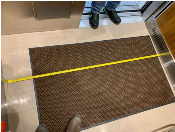
Photo 81 – Inside Dimensions of Elevator Car
