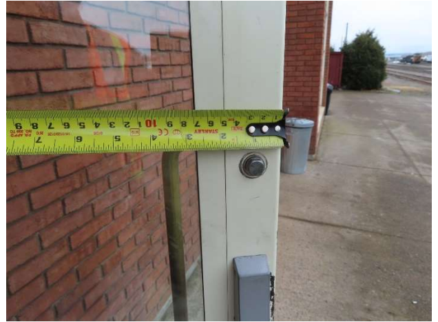
Photo 14 – Intercom height in a bedroom
