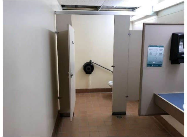
Photo 32 – Height of towel dispenser from finished floor
