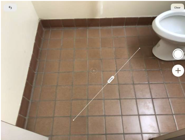
Photo 33 – General view of shower stall
