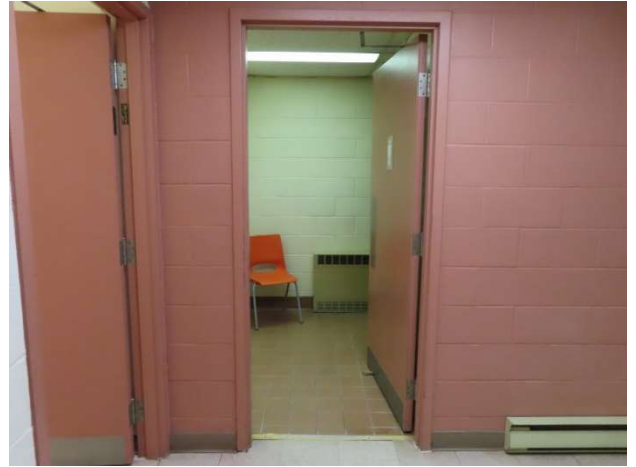
Photo 38 – Height of towel dispenser from finished floor
