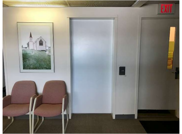
Photo 44 – Height of towel dispenser from finished floor
