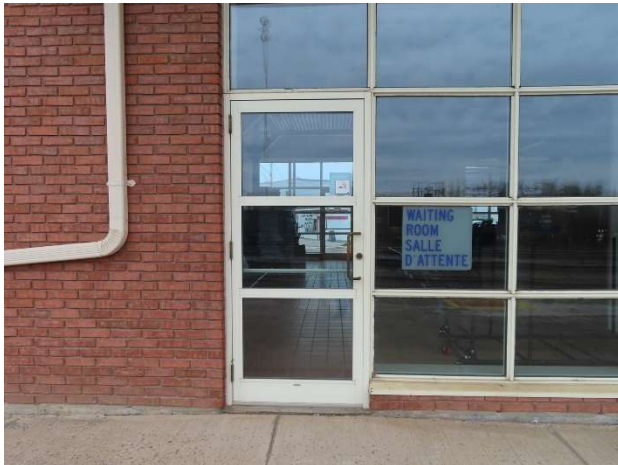
Photo 5 - Clear open door width of exterior door
