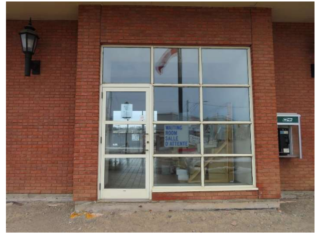
Photo 10 – Door opening mechanism height from ground
