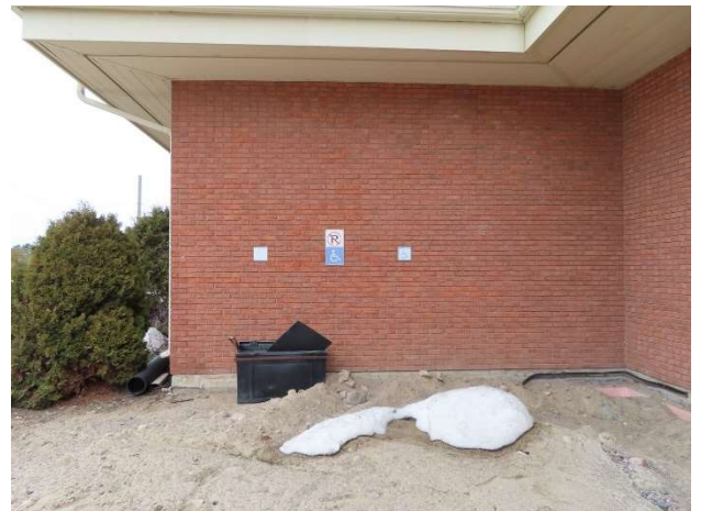
Photo 60 – Height of fire pull station from finished floor
