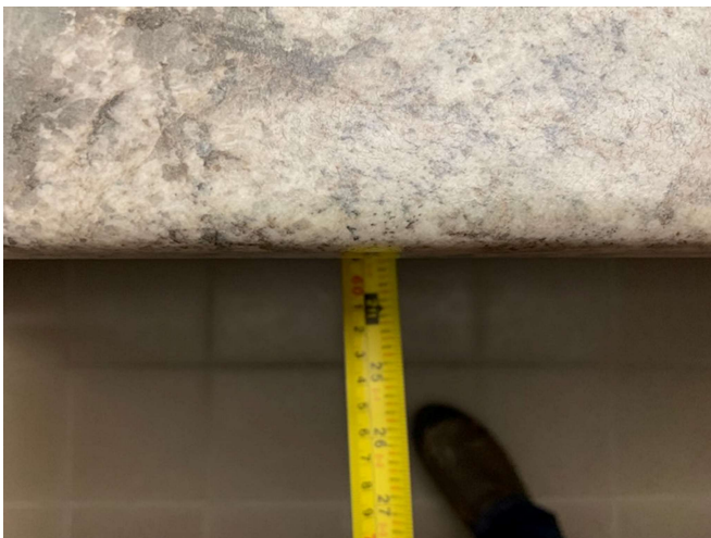
Photo 53 – Depth of floor space under lavatory
