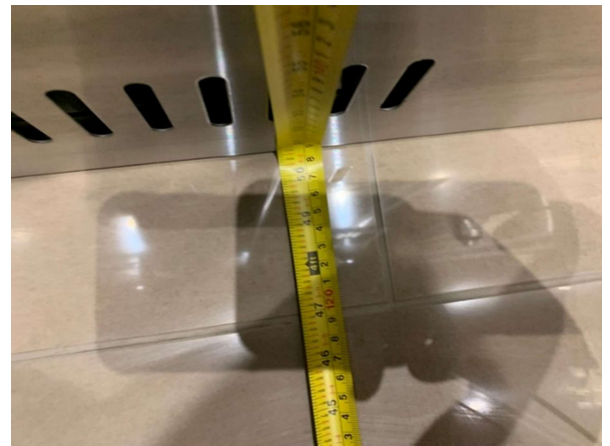
Photo 84 – Distance from Wall to Inside Face of Door (close-up measurement)
