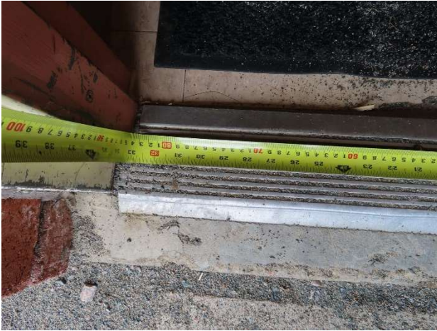
Photo 3 - Outdoor door of entrance vestibule
