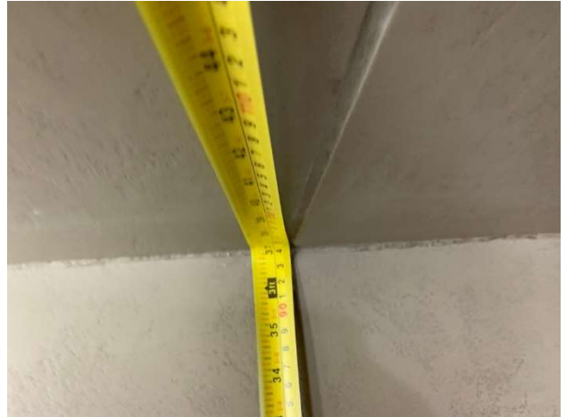
Photo 34 – Office Corridor - Clear width (close-up measurement)
