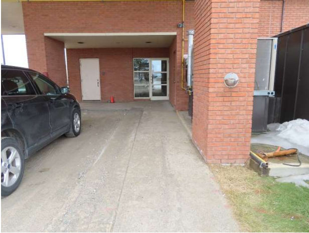
Photo 7 – General view of corridor and corridor entrance door
