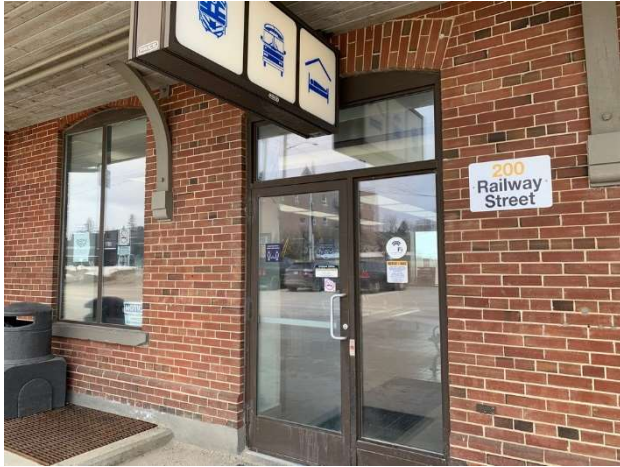
Photo 1 - General view of main entrance door – pull side
