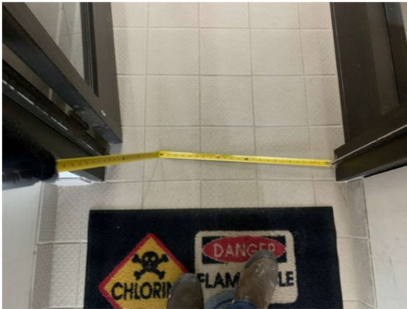
Photo 39 – Ticket Office Transition Door: Clear width of open door
