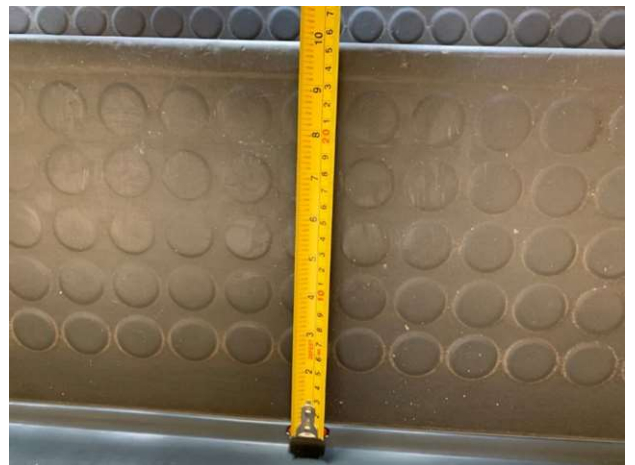
Photo 70 – Demarcated leading edge of the tread
