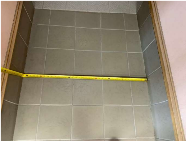
Photo 33 – Office Corridor - Clear width
