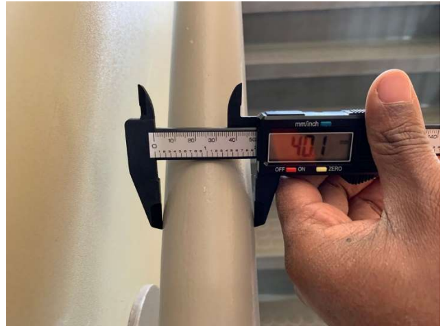
Photo 76 –Side Handrail: Diameter
