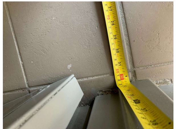
Photo 58 – Entrance Door opening width
