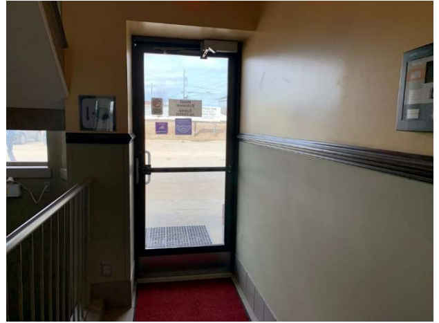
Photo 8 – General view of hotel entrance - Push side
