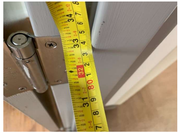
Photo 22 – Interior Door-Clear width of open door
