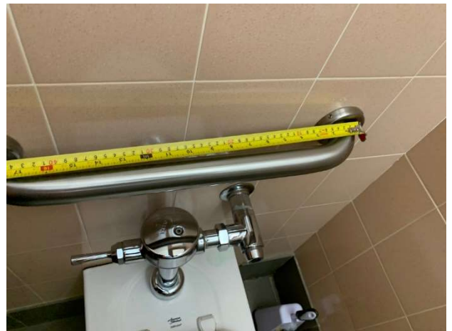
Photo 48 – Length of horizontal component of L-shaped grab bar
