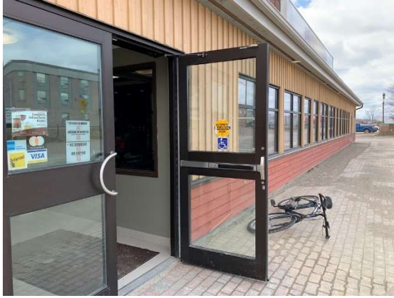
Photo 13 – General view of restaurant entrance outer doors
