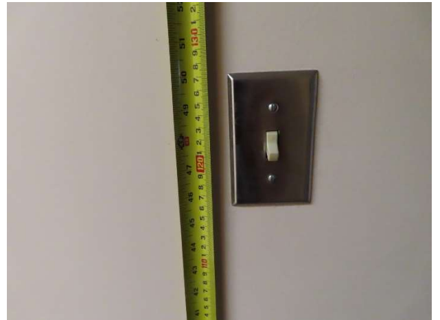
Photo 52 – Light switch height from finished floor
