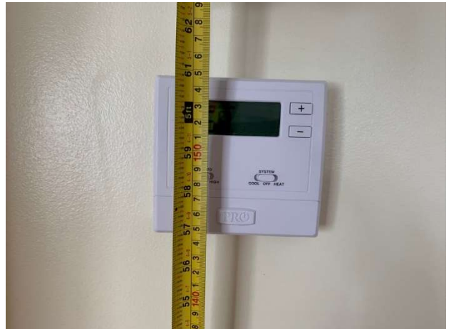
Photo 30 – Height at the thermostat
