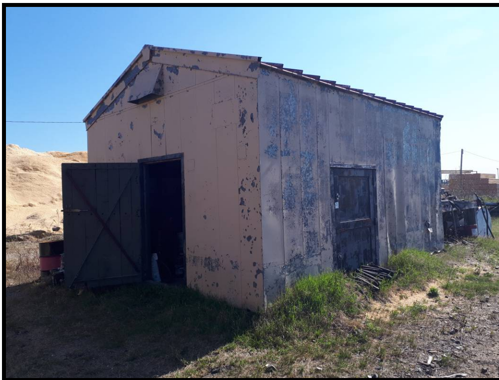
PHOTO # 4 Mechanical Department Shed – Hearst Site
