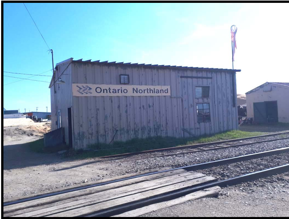
PHOTO # 5 Mechanical Building – Hearst Site
