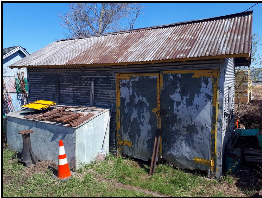
PHOTO # 2 Shed #2 – Hearst Site
