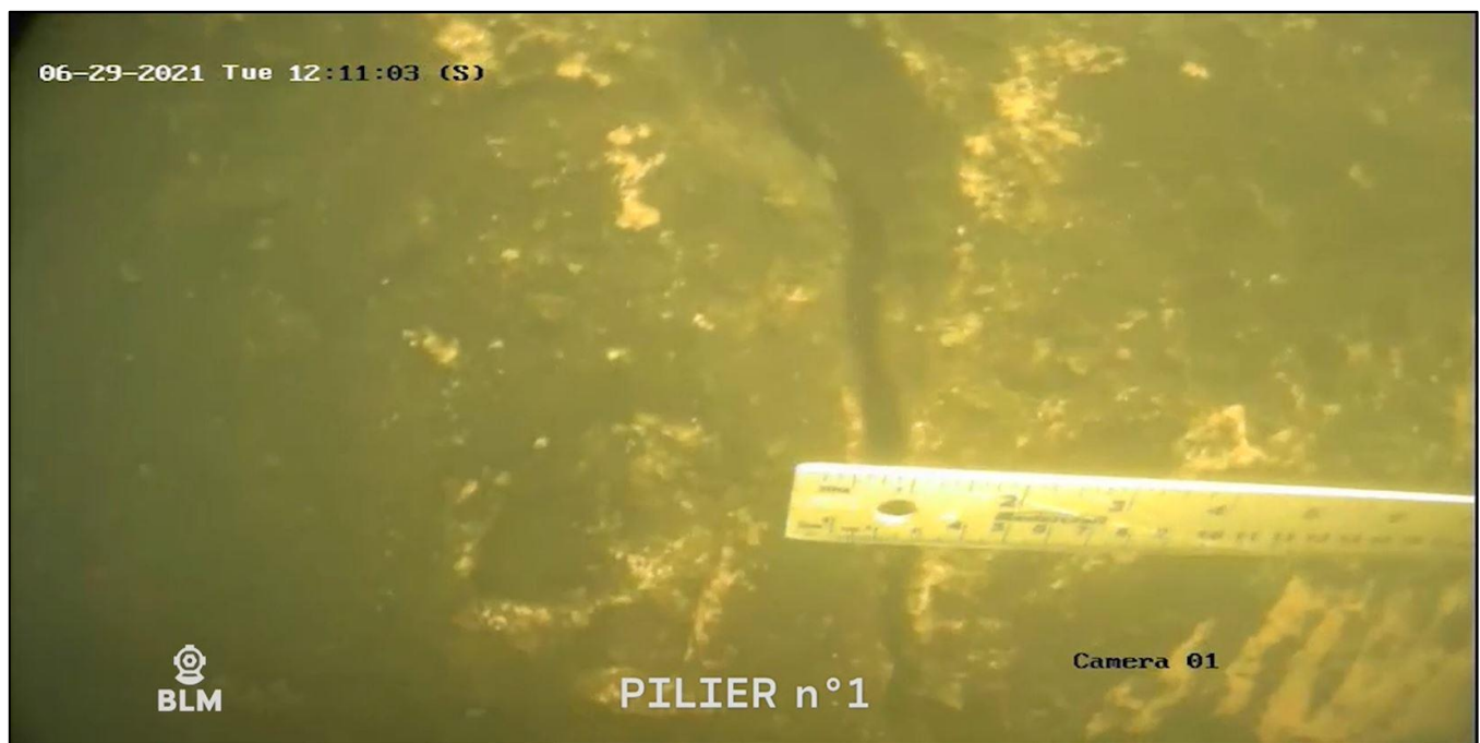
PHOTO 14 – PIER N°1 – CRACK 5 MM
