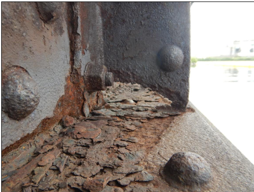
PHOTO 22 – CORROSION OBSERVED ON STEEL BEAM STIFFENERS
