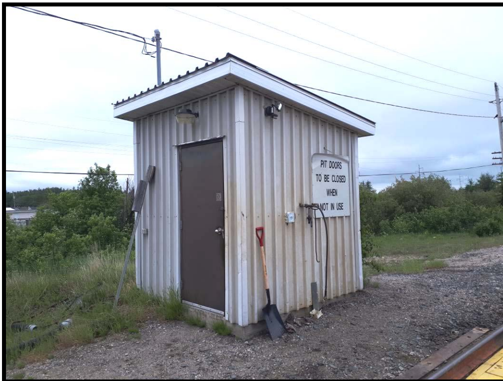
PHOTO # 17 Coach Sewer Dump Storage Shed – Cochrane Site
