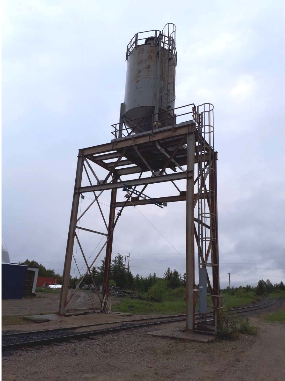
PHOTO # 7 Locomotive Sanding Tower – Cochrane Site
