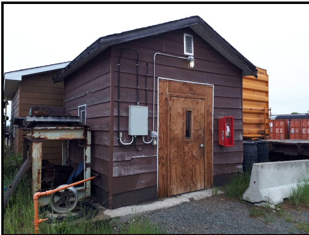
PHOTO # 13 Rip Track Fuel Shed – Cochrane Site
