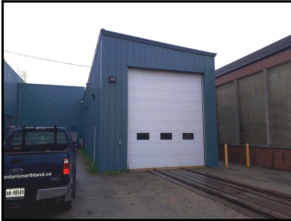
PHOTO # 5 Wheel Drop Pit Shelter – Cochrane Site
