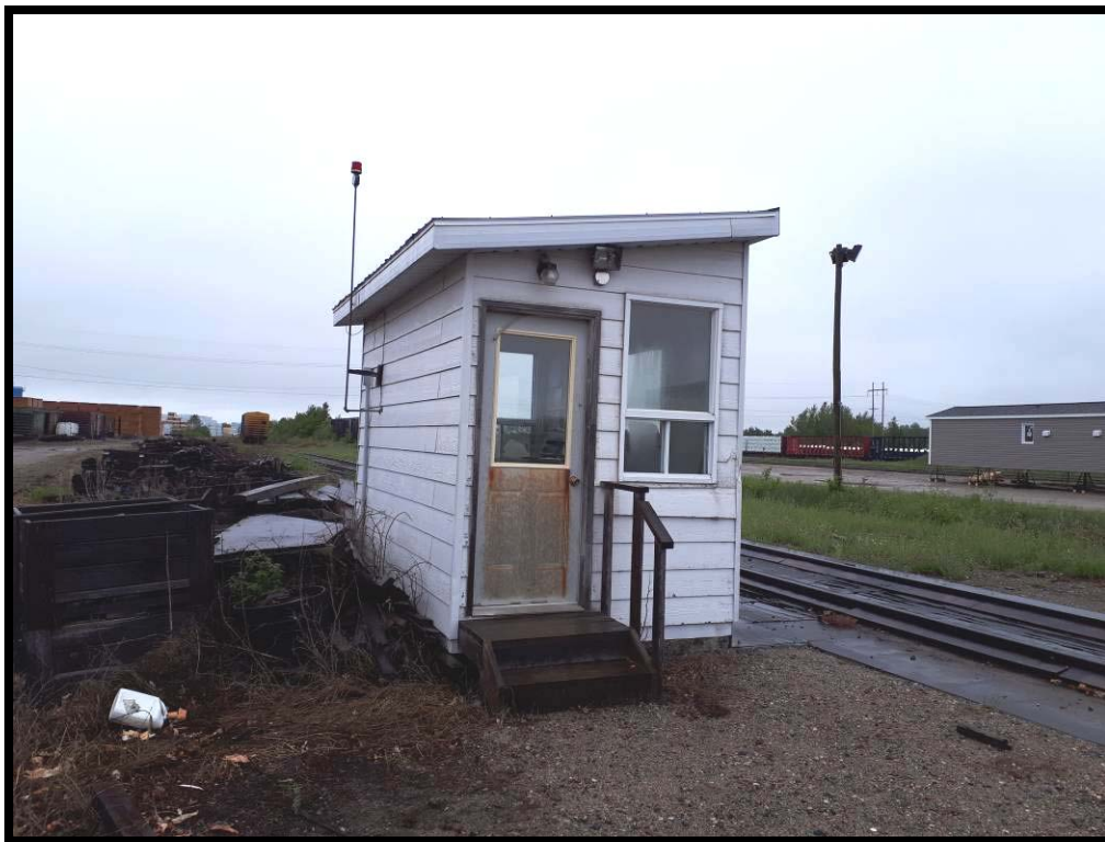
PHOTO # 9 Scale Building – Cochrane Site
