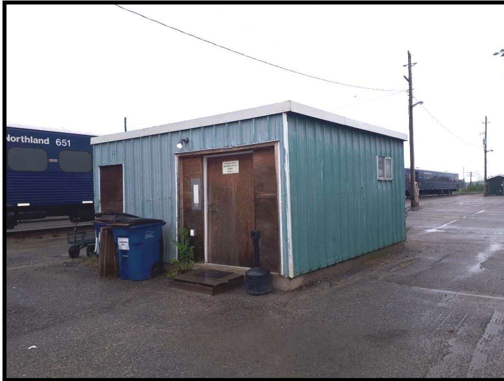
PHOTO # 3 Coach Cleaner Storage Shed – Cochrane Site
