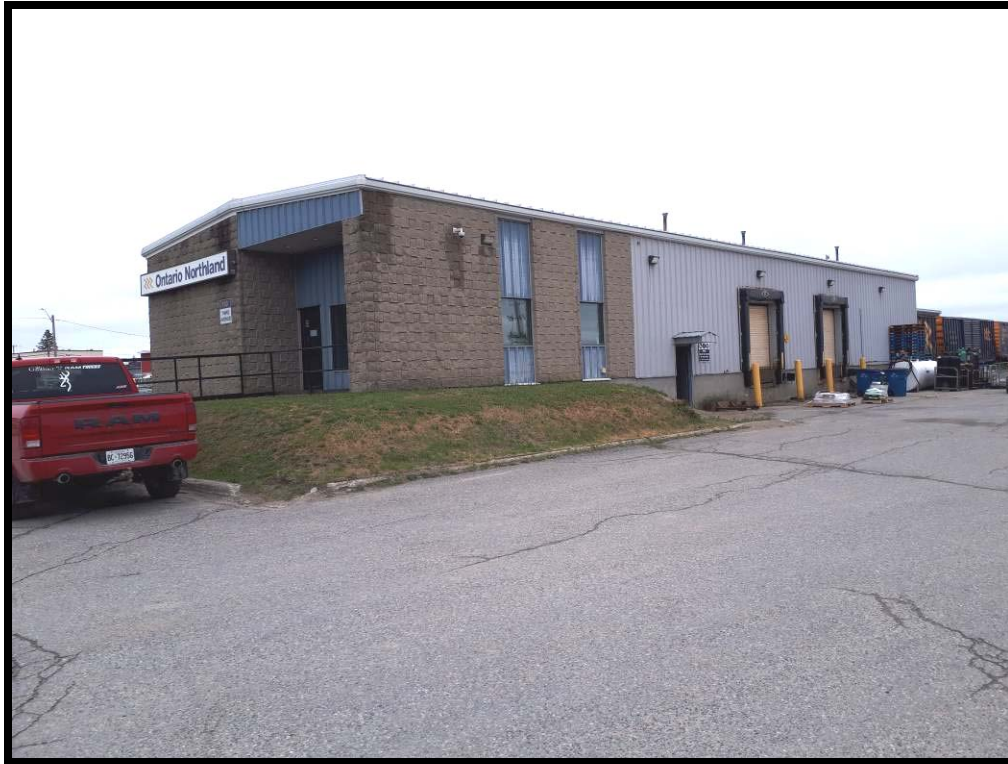
PHOTO # 18 Freight Shed – Cochrane Site
