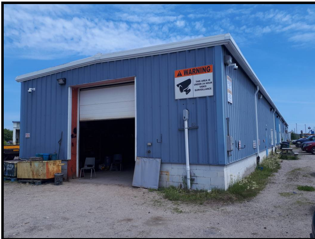
PHOTO # 23 Yard Office – Cochrane Site
