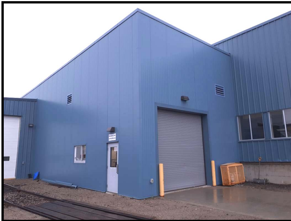
PHOTO # 6 Stores – Cochrane Site
