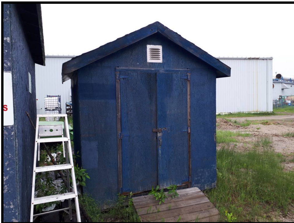
PHOTO # 11 Storage Shed #1 – Cochrane Site
