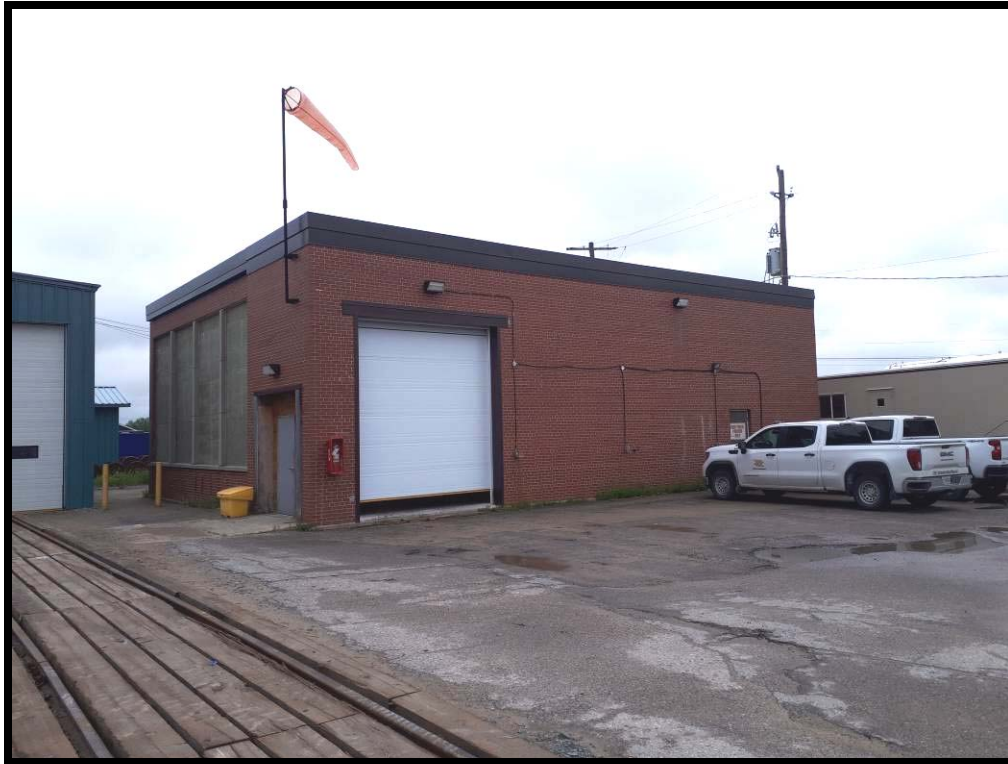
PHOTO # 8 Powerhouse – Cochrane Site
