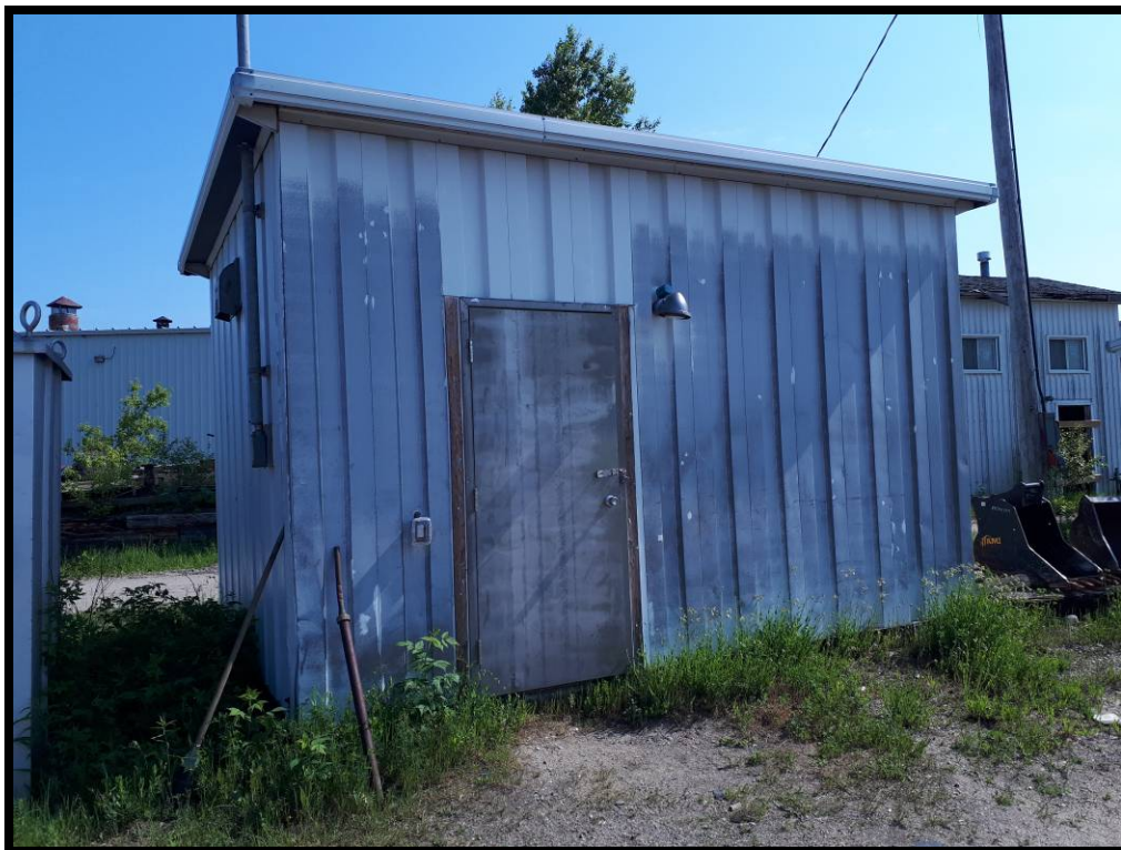
PHOTO # 21 MOW Water Shed – Cochrane Site
